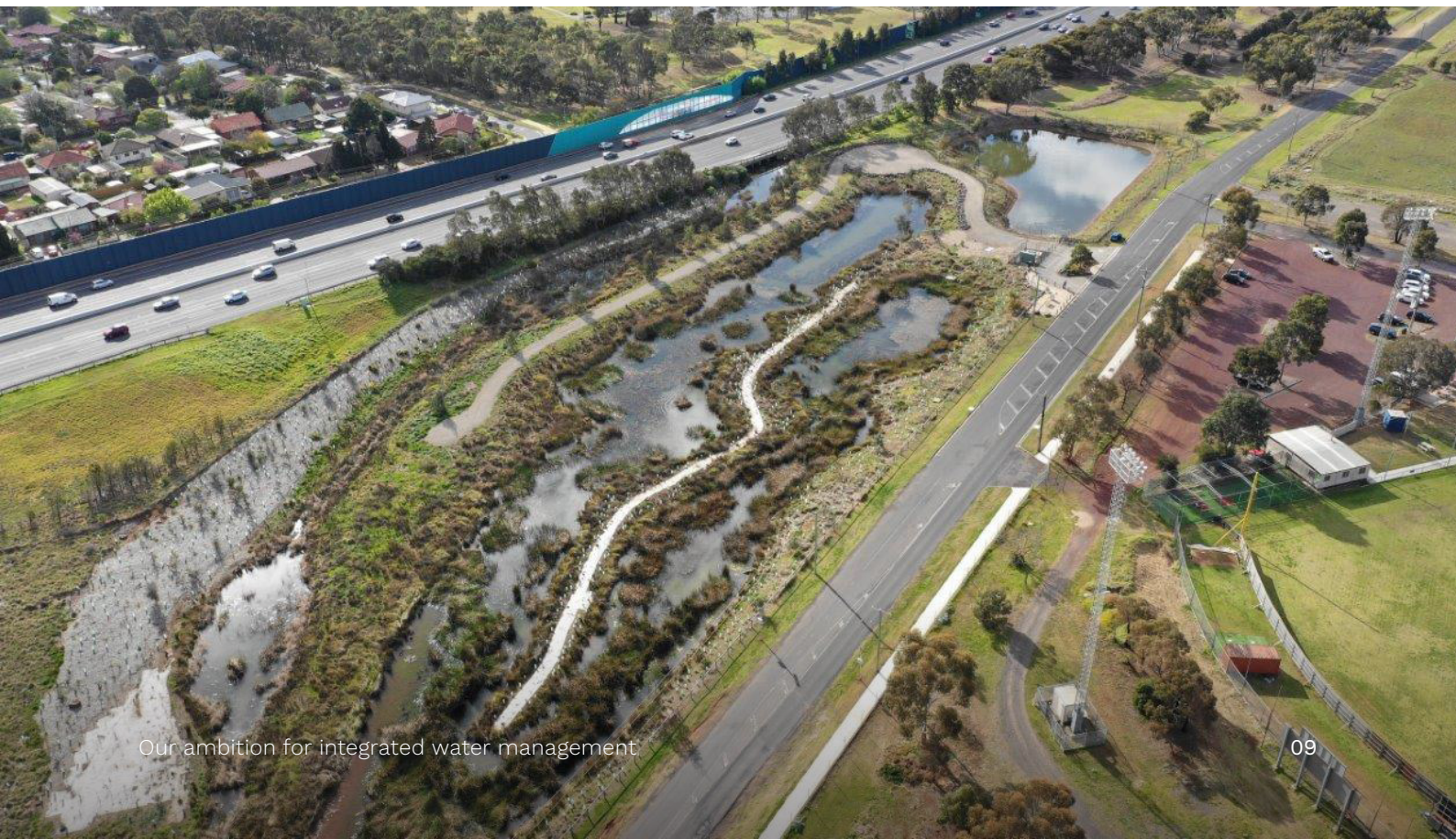
Image: Laverton Reserve, Laverton. Stormwater harvesting project.
