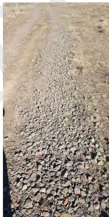
Low impact access track installed
