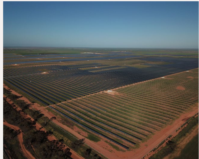
Figure 10. Kiamal Solar Farm supplies Zero Emissions Water program
