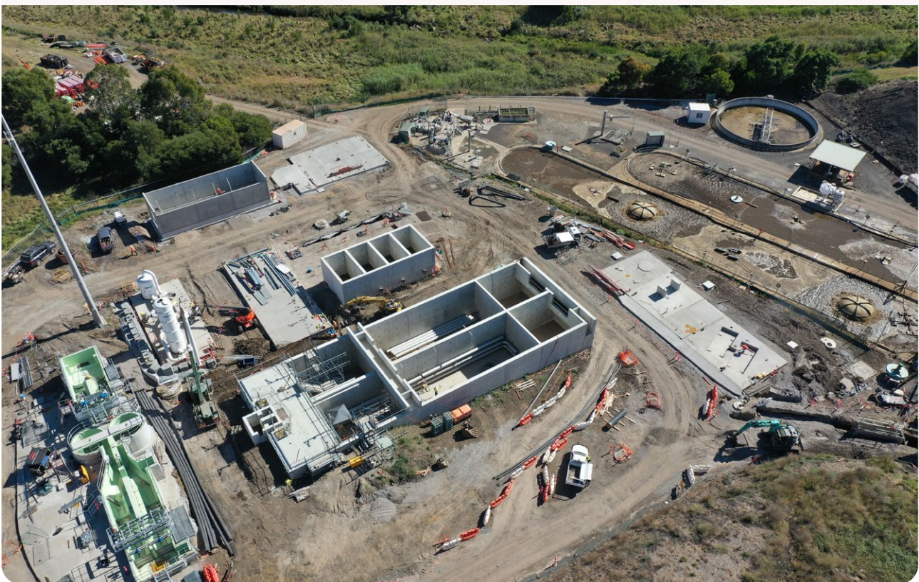
Figure 22. Gisborne RWP upgrade
