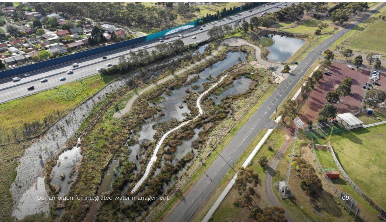
Image: Laverton Reserve, Laverton. Stormwater harvesting project.
