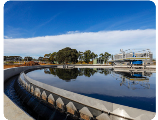
Melton Recycled Water Plant
