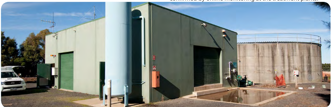
Romsey Water Filtration Plant
