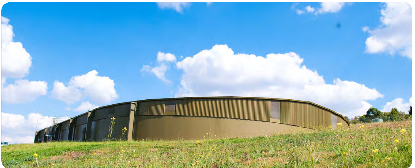
Drinking water storage tank near Bacchus Marsh (Merrimu supply system)
