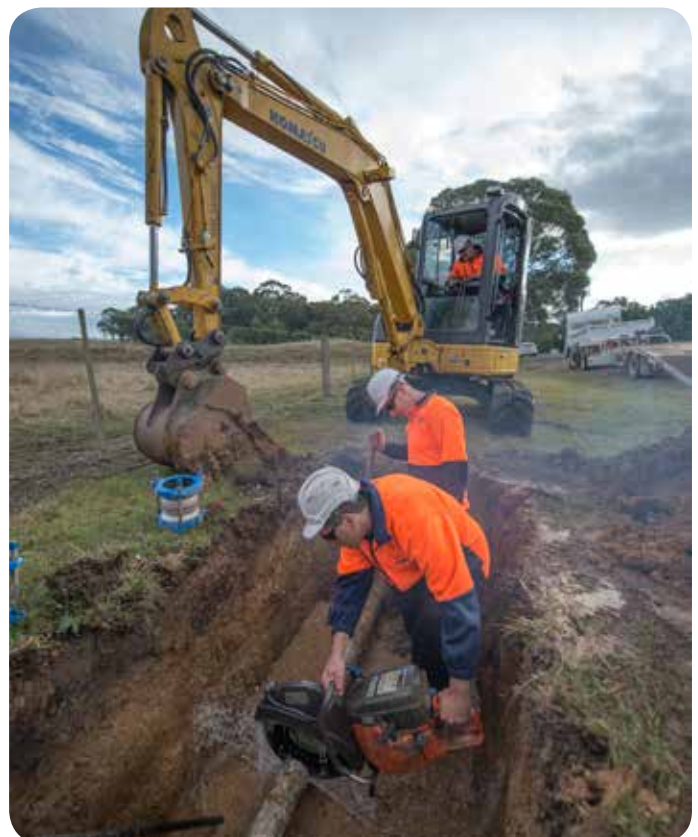
Emergency main repairs
