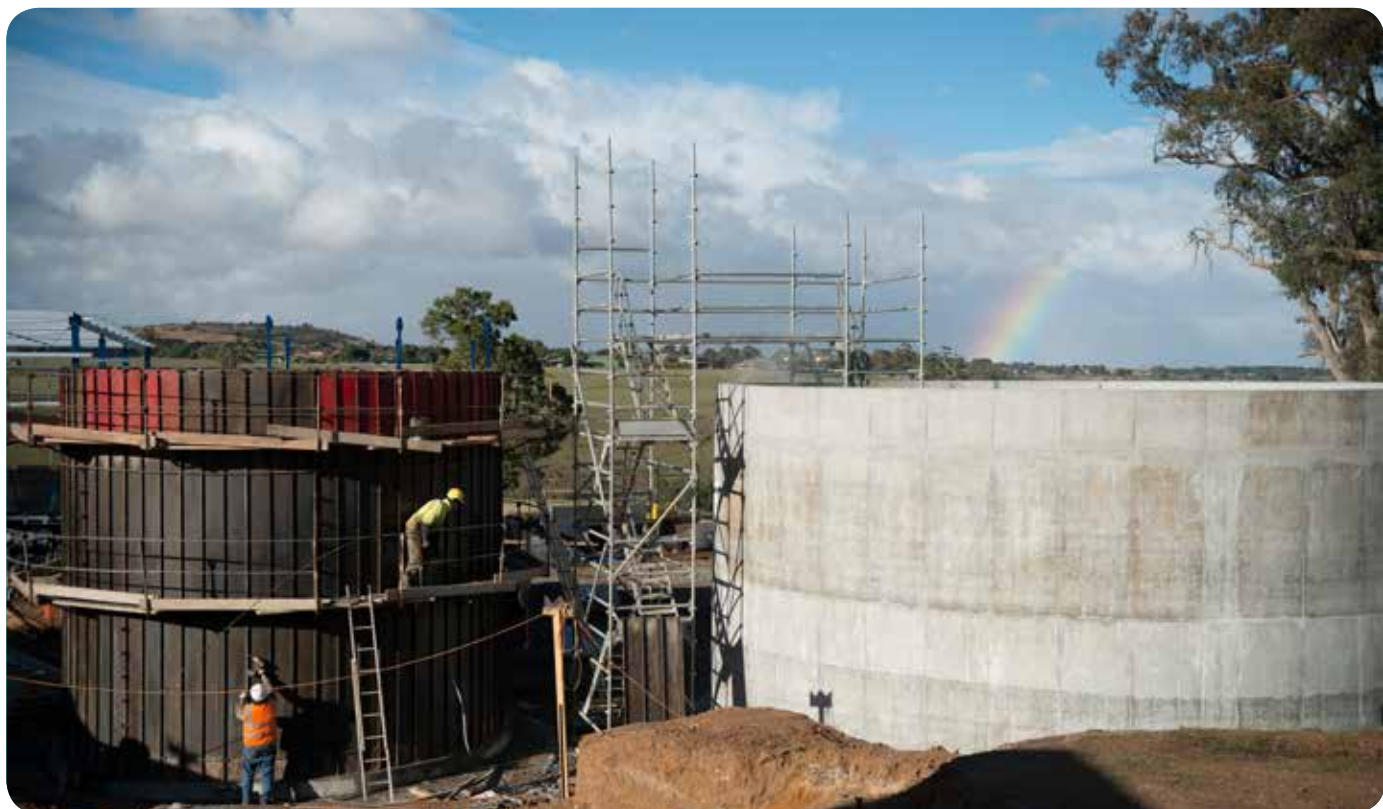
Tank construction work at Rosslynne WFP
